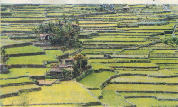
Constructing houses within the rice terrace area is a violation of the UNESCO WHS rules that they should be built along the border (buffer zones) so as not to destroy the landscape architecture. This cascade of the Hungduan Rice Terrace stretching along the one-hour mountainous road ride towards Banaue is called the Hapao Spider Web.
